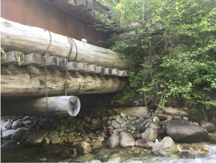
Left Bank Abutment
