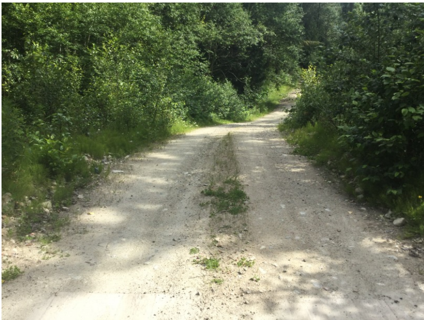
Left Approach Facing Away From Bridge
