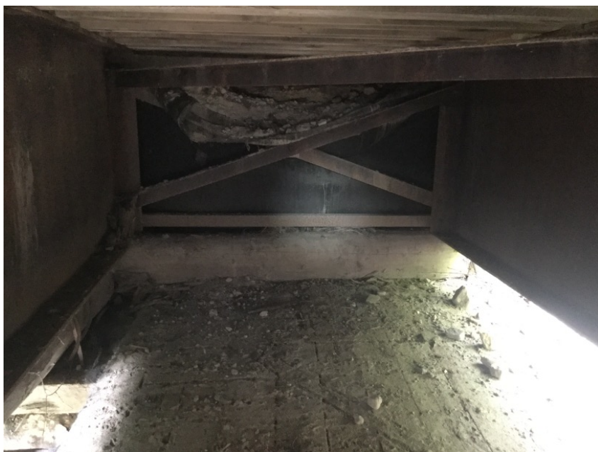
Right Bank Abutment
