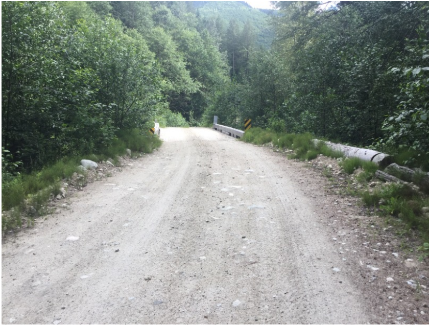
Right Approach Facing Bridge
