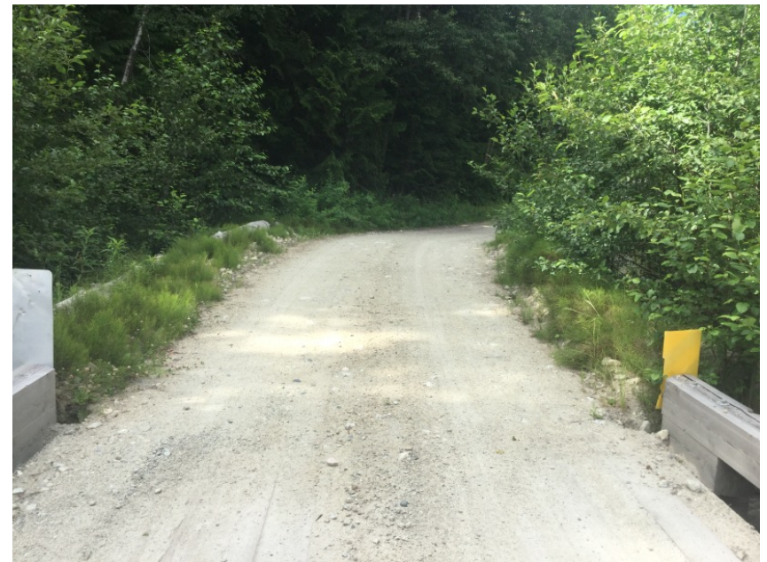
Right Approach Facing Away From Bridge
