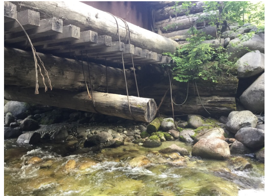
Left Bank Abutment
