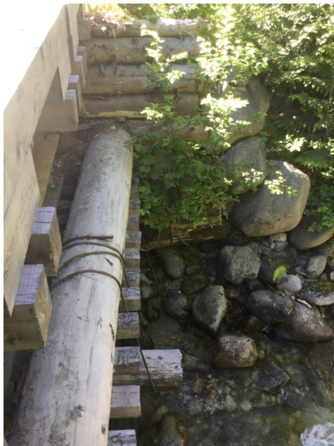
Sill Log Bearing on Old Bridge Deck & Log Crib
