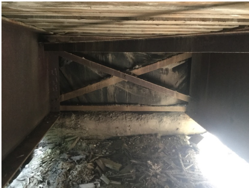
Left Bank Abutment
