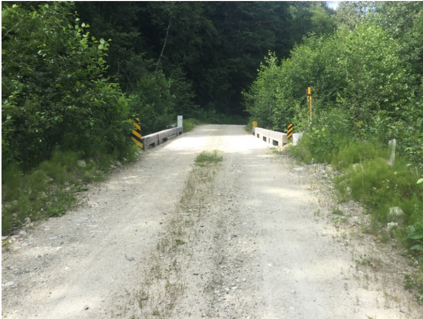
Left Approach Facing Bridge
